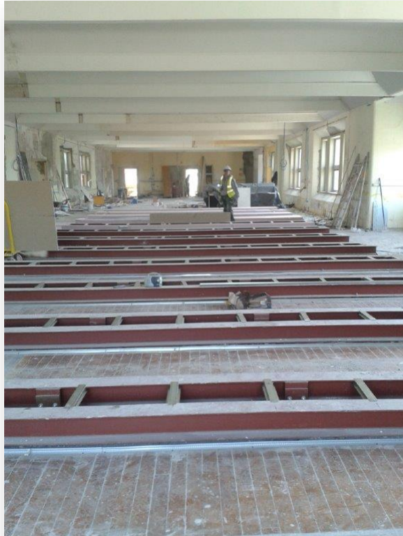
Steelwork support to new library shelving in S19
