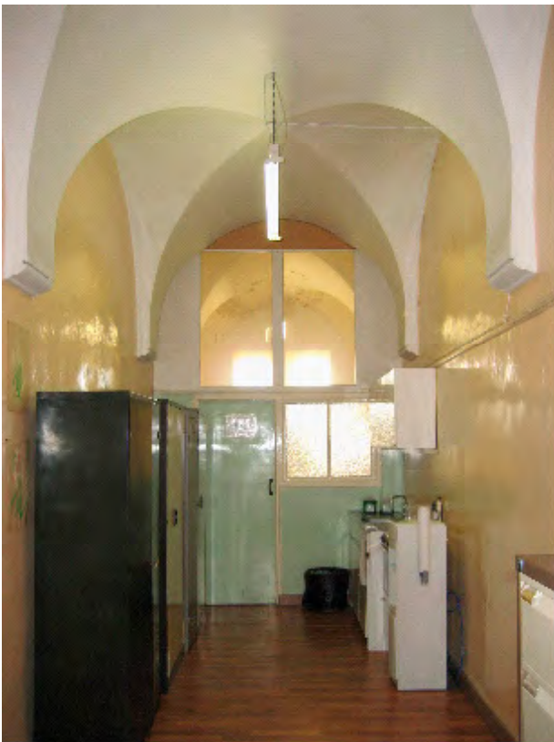
Vaulted ceilings in central spine extending from rear of front range
