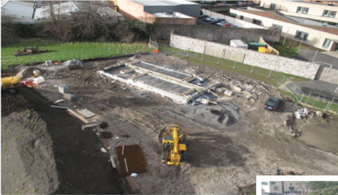
Figure 12: Energy Building construction of ground floor slab.
