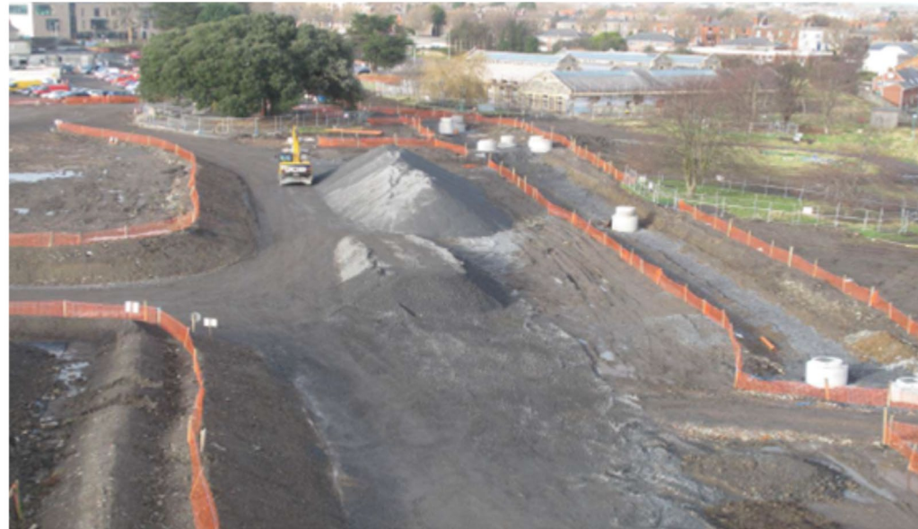
Figure 1: Haul Road and drainage manholes constructed along Ivv Avenue.
