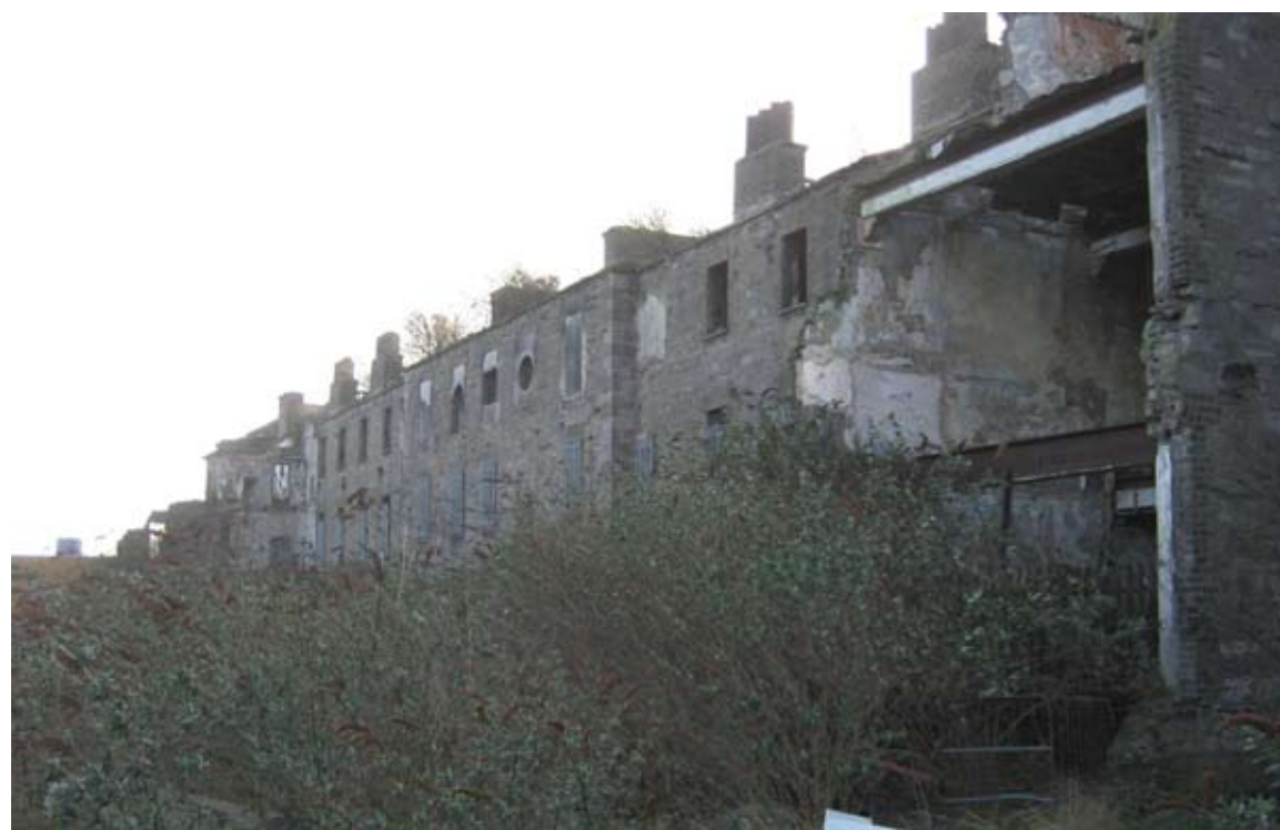
North elevation of surviving southern wing—showing the truncated western return wing of the original quadrangle complex. This photograph also illustrates the poor condition of this structure.
