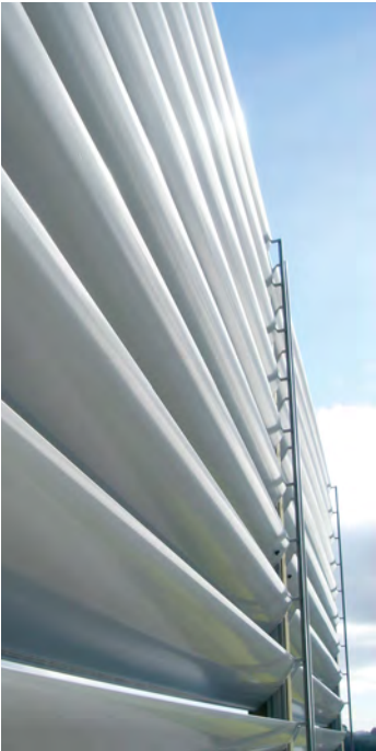
Examples of rooftop screening for mechanical equipment
