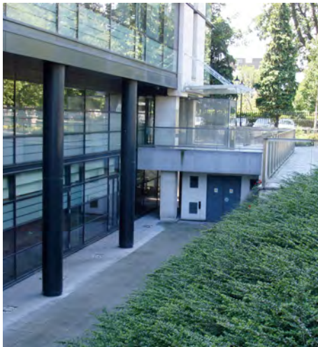
Pulling away the ground to allow light to enter lower levels.
