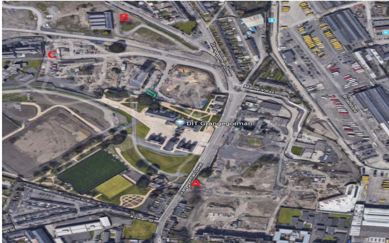
Figure 1: Dust Monitoring Locations, A B and C.
